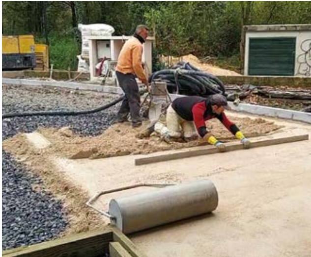
Drainage floor installed in the outdoor area.
