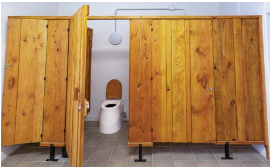
Dry toilets installed.
