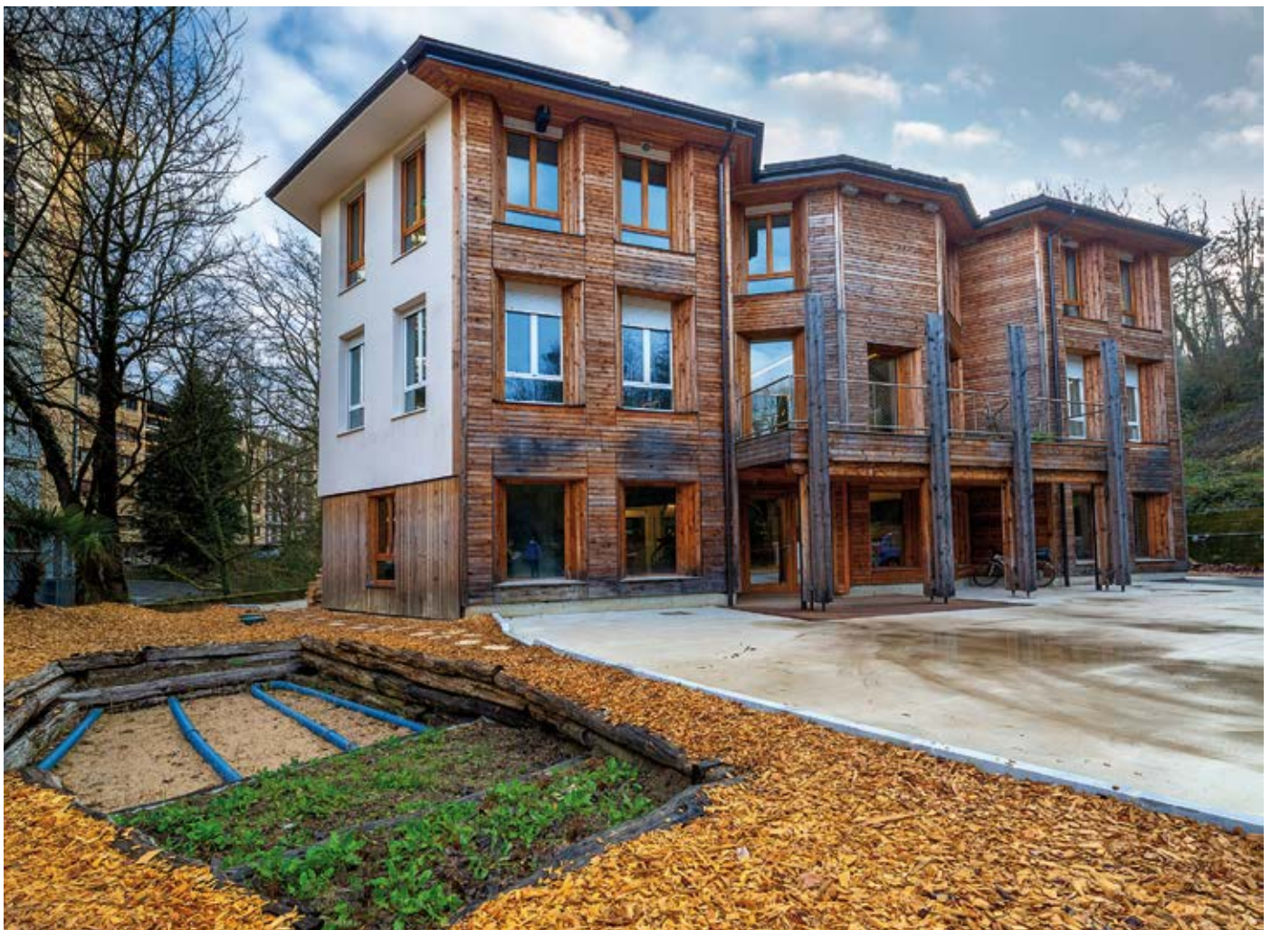
View of the Natur Eskola from the outside after the intervention was completed.
