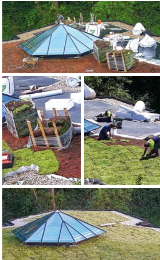
Green roof implementation process.
