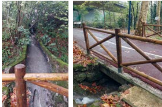
Side ditch to collect runoff water from the A8 motorway.
