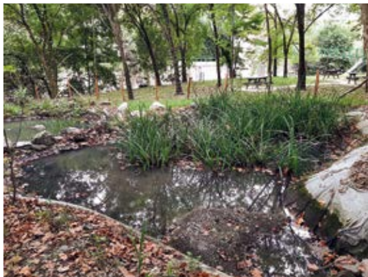
Side ditch to collect runoff water from the A8 motorway.
