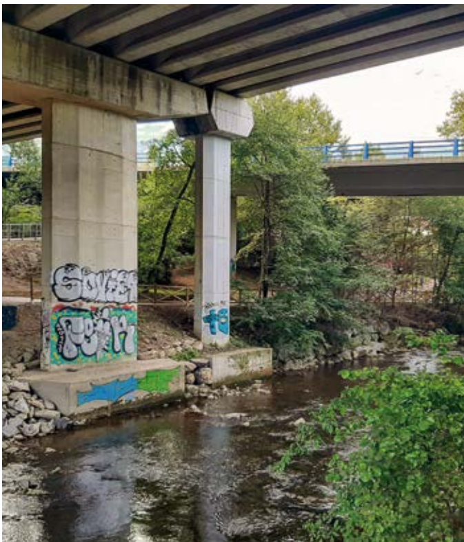
Viaduct where some of the interventions are located.
