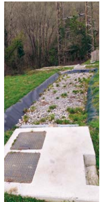
Phyto-purification system and grease separation tank.
