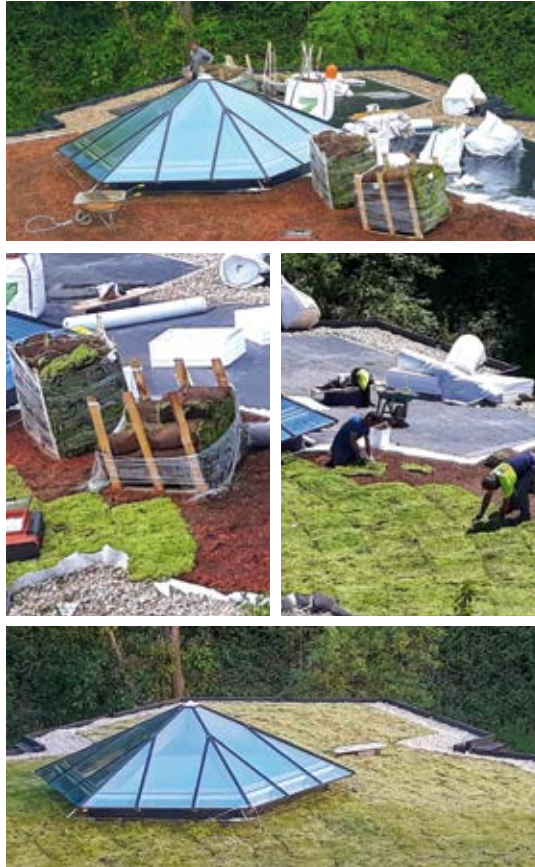
Green roof implementation process.
