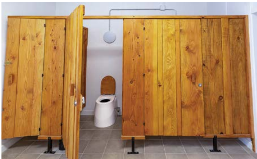
Dry toilets installed.
