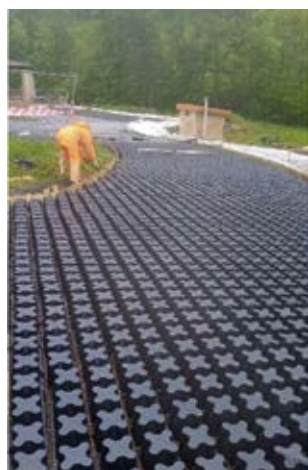
Perforated concrete slabs used for traffic road bases.
