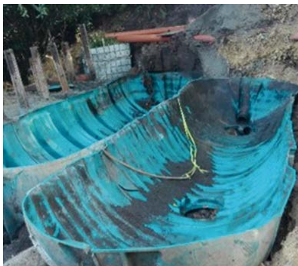
Placement of the two halves of the septic tank to install the purification system, after it was emptied and cut into two.
