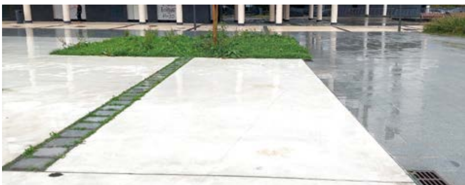
Drainage strip (left) after completion of the work and conventional rainwater collection pit (right).
