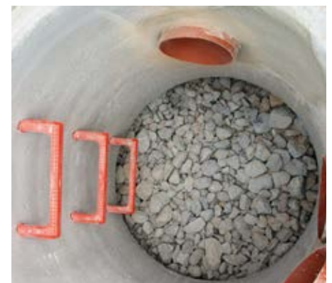
Access chamber upon completion of the work.
