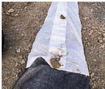
Green ditch construction process.
