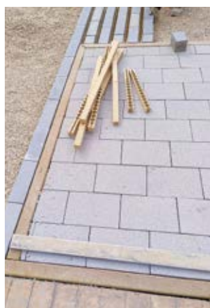
Continuous porous concrete flag stones for pedestrian pavements.
