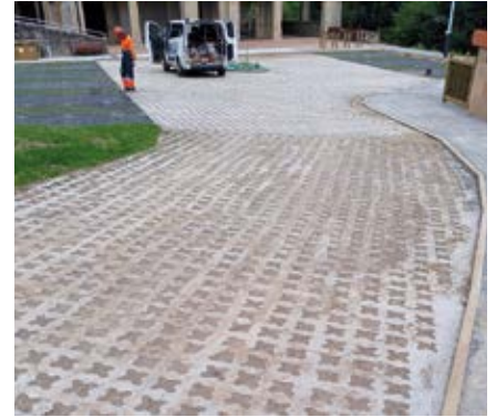
Concrete cells for traffic road bases.
