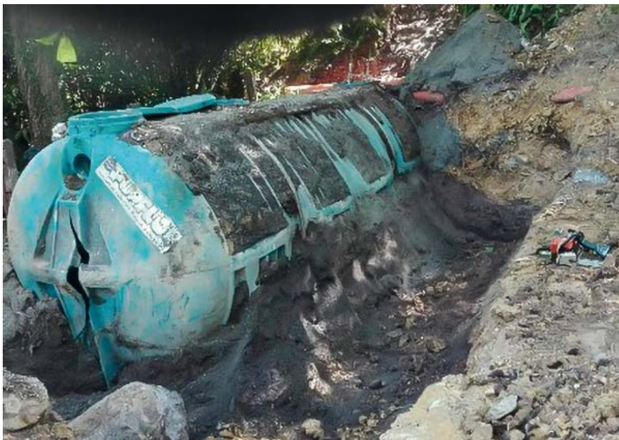
Excavation next to the pre-existing septic tank.
