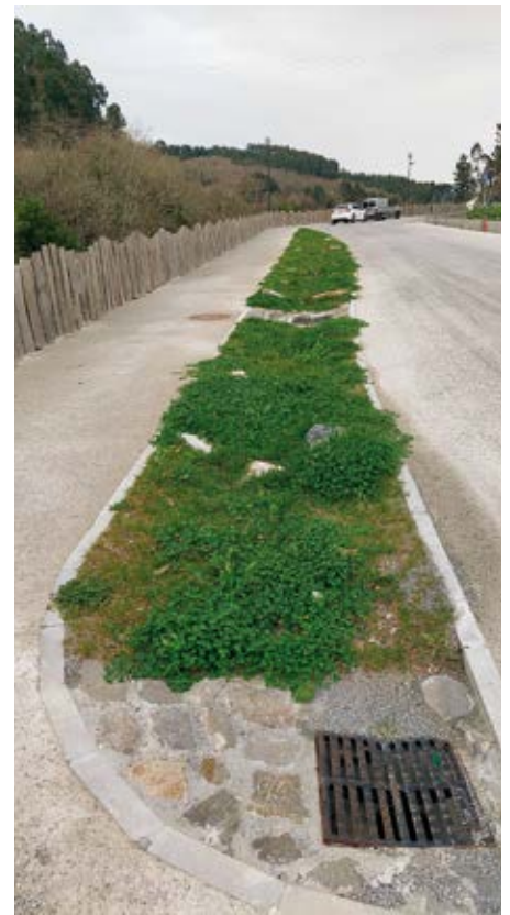
Green ditch six months after completing the work.
