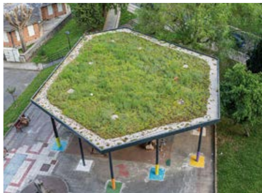
Images showing the Laubide green roof installation process.
