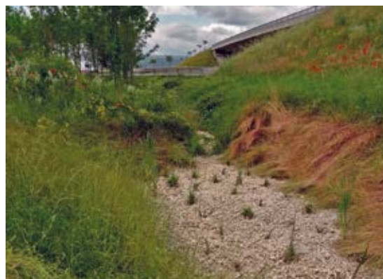
Green filter with gravel bed and aquatic vegetation.
