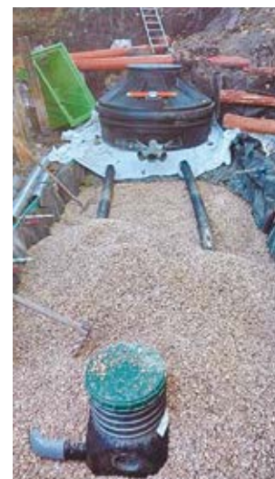
Installation of equipment and backfilling of wetlands once the two parts of the septic tank were sealed.
