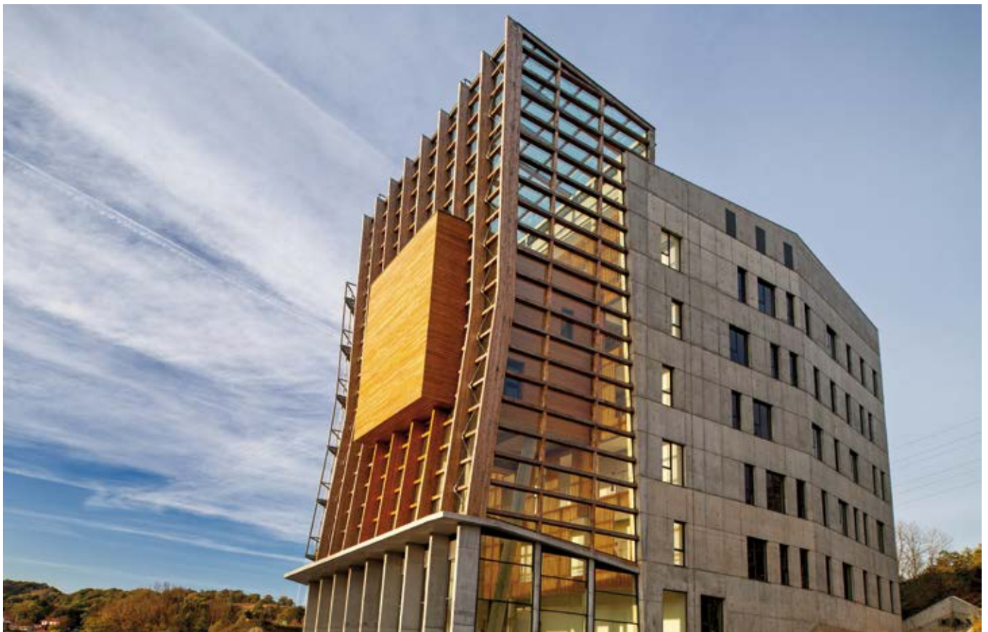
Exterior view of the ENERTIC building.
