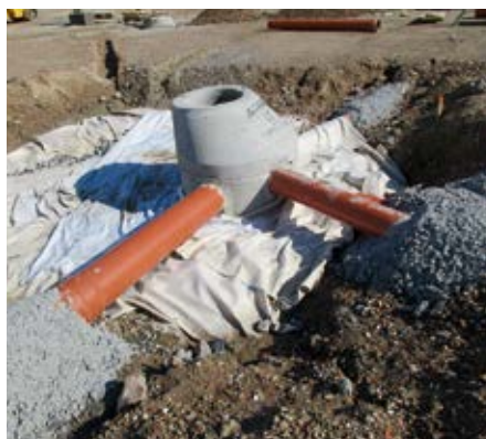
Access chamber under construction.
