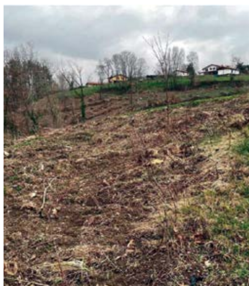
Clearing and preparation of plots.
