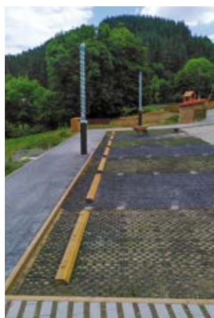
Recycled polypropylene cells filled with different shades of gravel for parking spaces.
