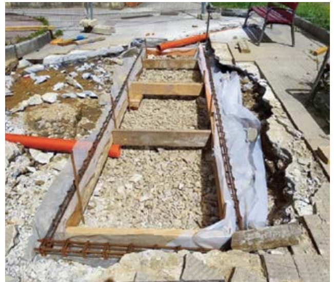
Excavation and laying of geotextile.
