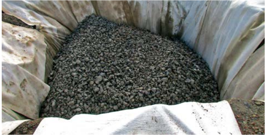
6 m deep gravel infiltration column to ensure drainage.
