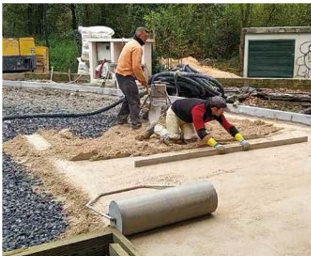
Drainage floor installed in the outdoor area.
