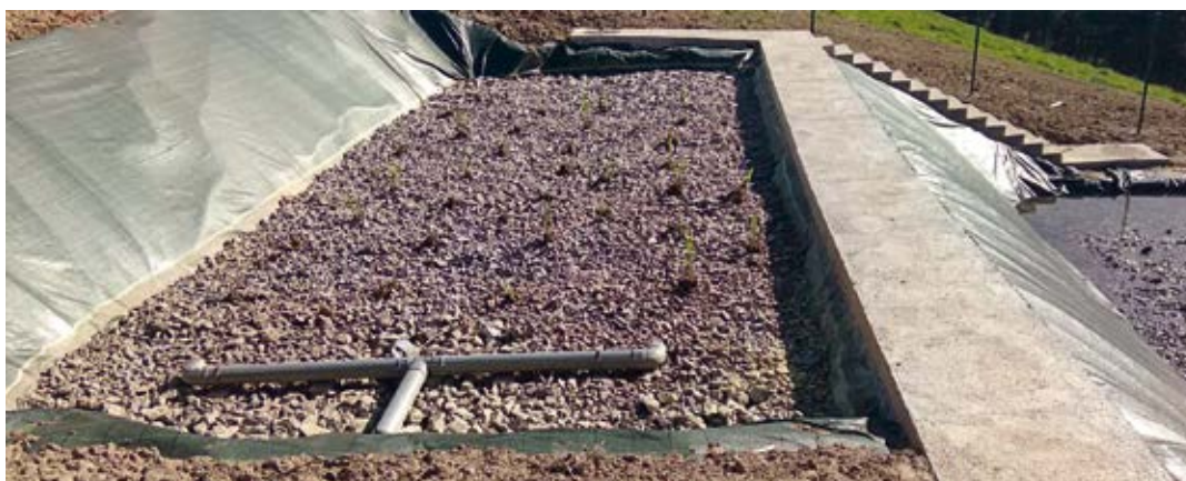
Lower basin of the constructed wetland, showing the gravel filtering substrate with different grain sizes and a thickness of 60 cm, in which the aquatic vegetation is planted.
