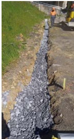
Construction of the drainage ditch (photo on the left) . Drainage ditch with vegetation after completion of the work (photo on the right).
