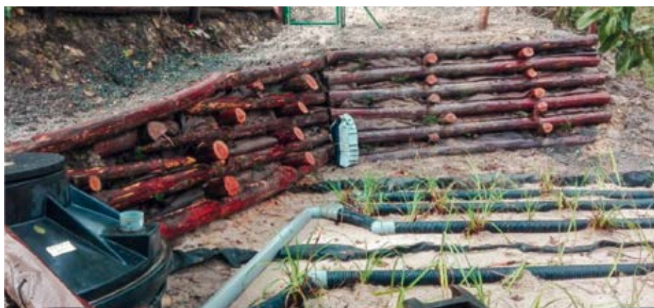
Construction of a permeable wall to stabilise the slope.
