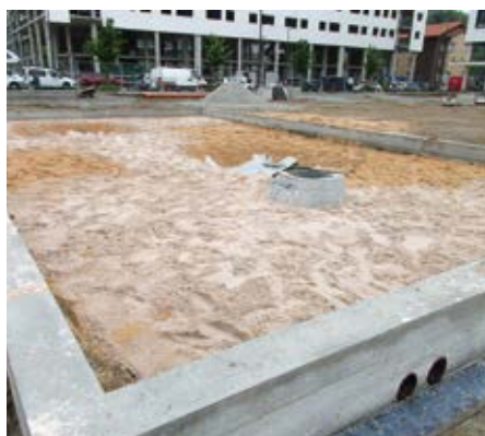
Rain garden construction process.
