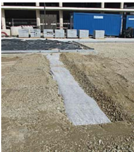
Drainage strip construction process.
