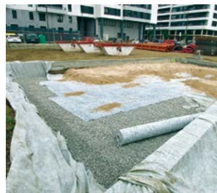
Rain garden construction process.
