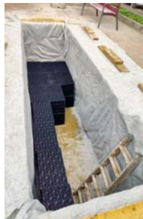
Backfill with drainage cells and gravel.
