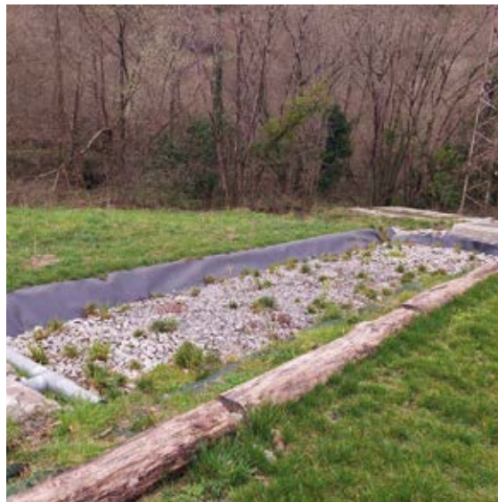
Phyto-purification system and grease separation tank.
