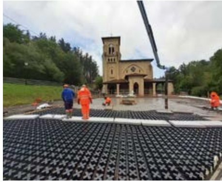
Perforated concrete slabs used for traffic road bases.
