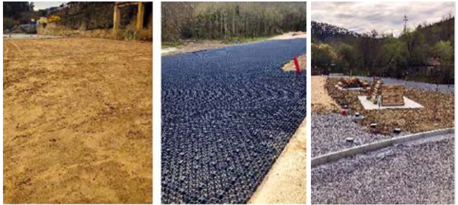
Installation of polypropylene cells.
