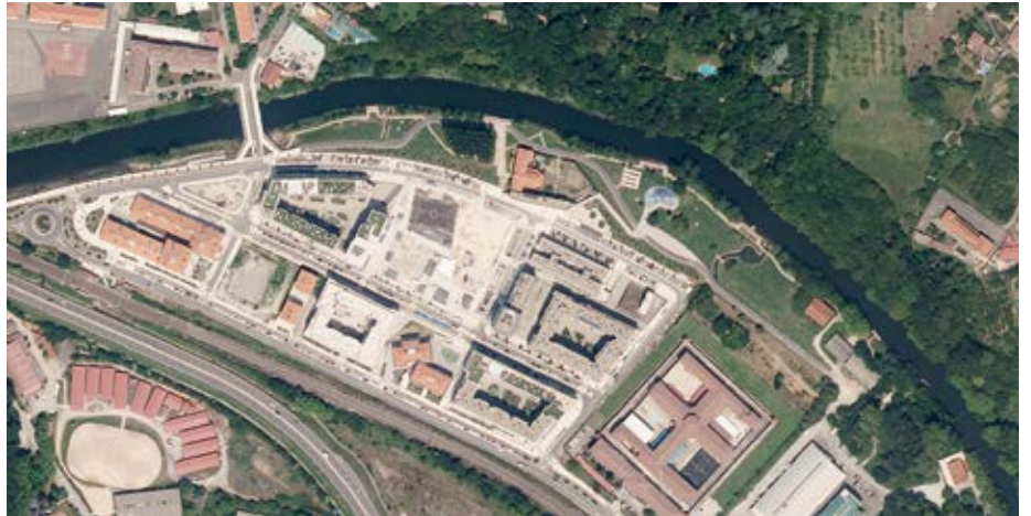
Aerial view of the area in 2022.
