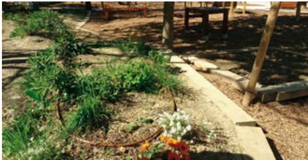
Drip irrigation connected to the rainwater harvesting system.
