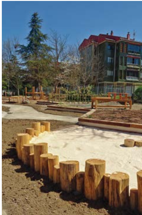
Topsoil in depaved areas.
