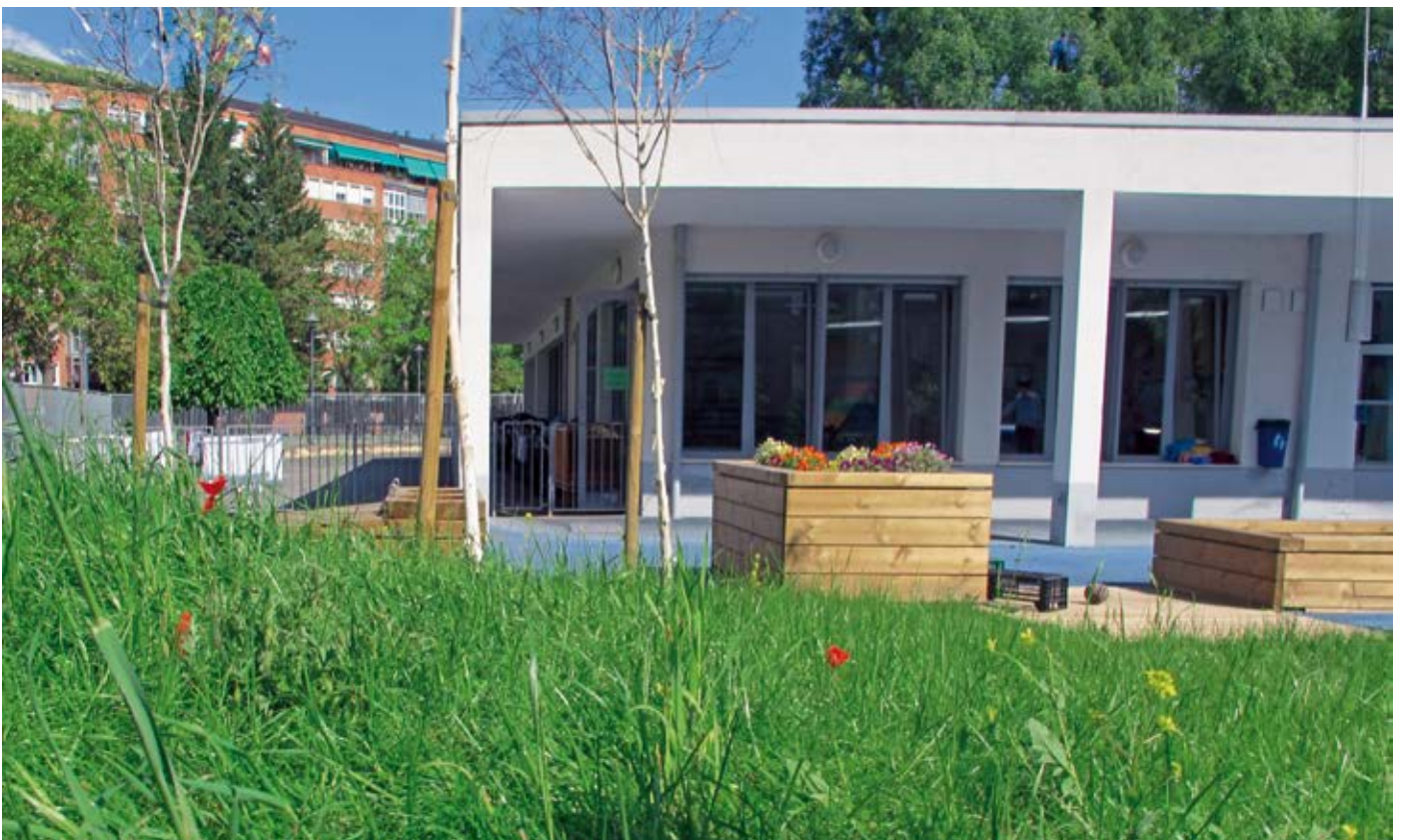
General view of the playground after the work was completed.
