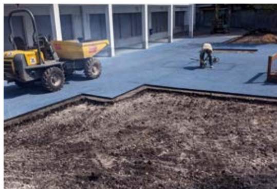
Initial condition of the playground and works to remove the paving.
