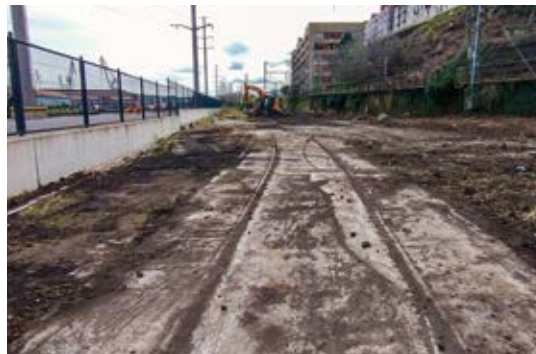
Appearance of the plot after clearing and levelling the land.
