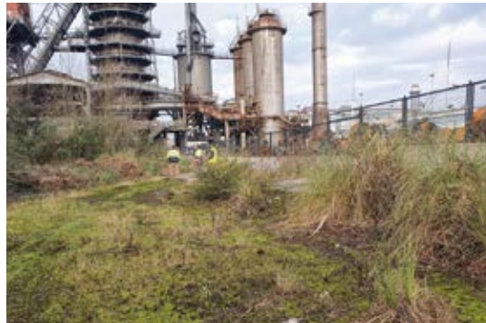
Appearance of the plot before the intervention.
